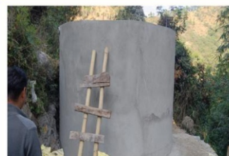
3. Percolation Well (Dia= 3.00 M & DEPTH=4.50 M) With Circular Pump House (DIA= 3.24 m & HT.= 2.70 m) – (Colour Palette Design Sample)
