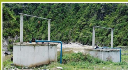
3. Percolation Well (Dia= 3.00 M & DEPTH=4.50 M) With Circular Pump House (DIA= 3.24 m & HT.= 2.70 m) – (Colour Palette Design Sample)
