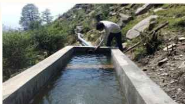
Construction work at FIS Khalagwad Nallah to Tikroo on 08.05.2024
