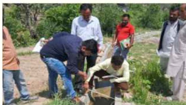
Construction work at FIS Shani Mandir Panchakkar under BPMU Gohar on 06.06.2024
