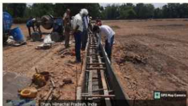
Construction work at LIS Dhan under BPMU Jawali on 18.06.2024
