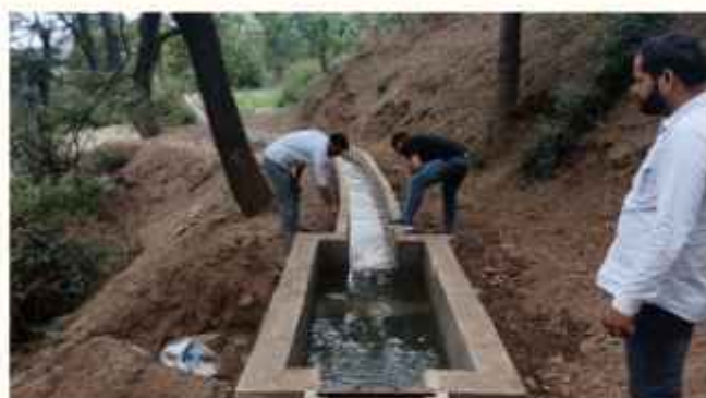
Construction Work at FIS Giri to Khadar under BPMU Nahan on 10.06.2024
