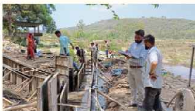
Construction Work at FIS Channour under BPMU Dehra on 07.05.2024
