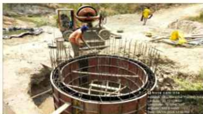
Construction Work at LIS Mandholi under BPMU Una on 25.06.2024
