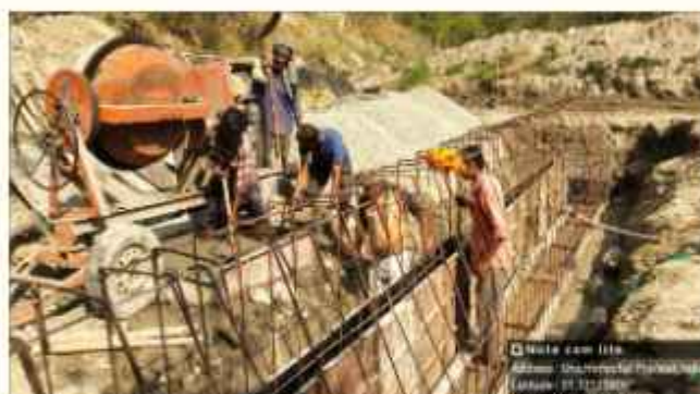
Construction work at LIS Mandholi under BPMU Una on 29.05.2024
