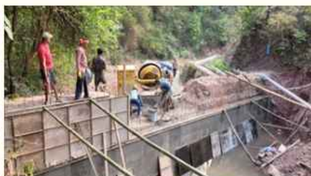
Construction Work at FIS Kothi Batala Jeora under BPMU Bilaspur on 24.05.2024
