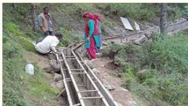
Construction Work at FIS Kandlu to Bithri under BPMU Gohar on 29.09.2024
