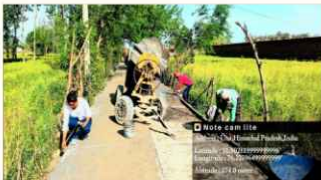
Construction Work at FIS Kandlu to Bithri under BPMU Gohar on 29.09.2024
