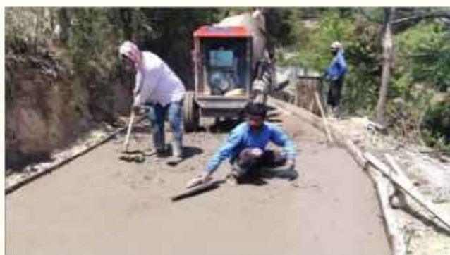
Construction Work at FIS Meru under BPMU Chamba on 24.09.2024
