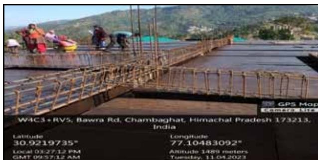
Beam reinforcement at FTC Solan.
