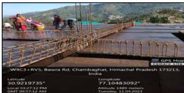
Beam reinforcement at FTC Solan.
